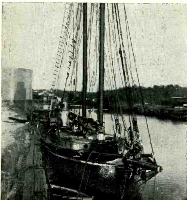
A typical tough antenna installation problem.
